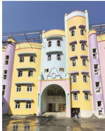
Current Site Picture Near Completion
